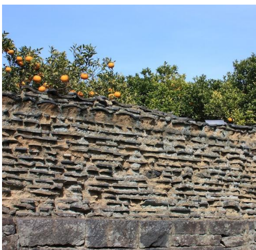
Mud wall and Summer Orange
